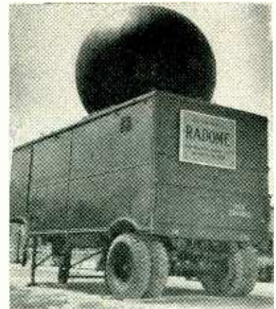
This new inflatable rayon radome displayed at Fort Monmouth is self-supporting and therefore requires less radar-opaque material. Once inflated, it requires only as much pressure as that generated by the conventional tank-type vacuum cleaner. Its purpose is to protect the pedestal and antenna of radar set against Arctic cold
